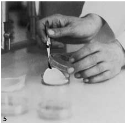
Placing the membrane filter on a nutrient pad after filtration
